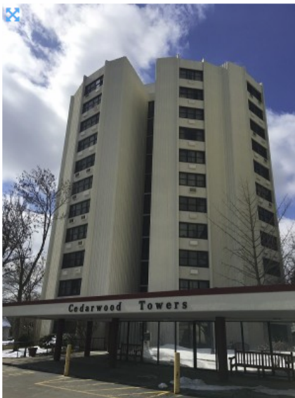
The 206-unit Cedarwood Towers in Rochester, N.Y., is undergoing a major rehabilitation by Community Preservation Properties and Rochester's Cornerstone Group.
