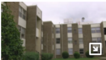
Every single one of the 216 units is going to be completely renovated.
