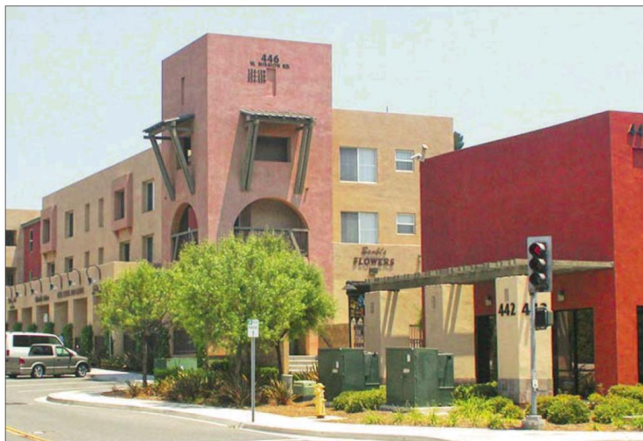
Paseo Del Oro in San Marcos is one of several affordable housing projects being renovated.
