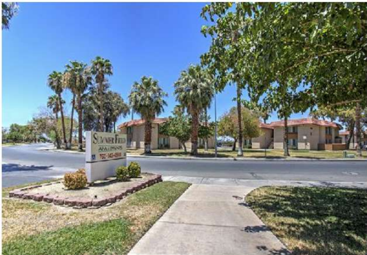
Photo taken prior to renovation work
